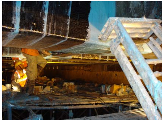
Fig. 8 Application of FRP laminates to the T-Beam at the site
