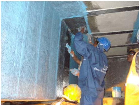
Fig. 8 Application of FRP laminates to the T-Beam at the site
